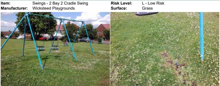
Finding: The soil is thin and there are rocks just under the Action: Provide an appropriate safety surface surface which will not provide the required impact protection
