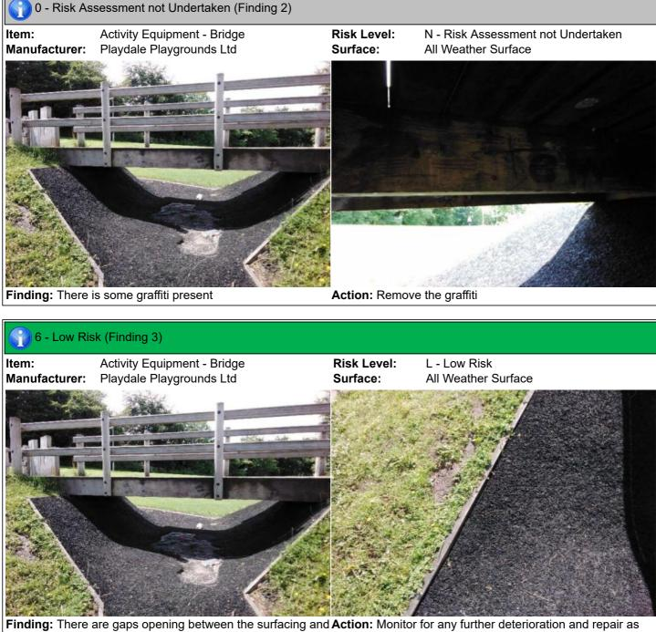
**Finding:** There are gaps opening between the surfacing and **Action:** Monitor for any further deterioration and repair as the edging surround or between the joints in the surfacing required
