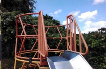
**Finding:** This item has no slide bar fitted as required by BS **Action:** Monitor - No remedial work recommended EN 1176 Part 3
