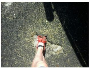
**Finding:** The surfacing around the item is damaged and is creating a potential trip hazard
