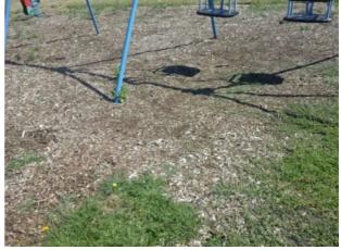
Finding: The loose fill safety surfacing has become compacted and degraded to mulch
