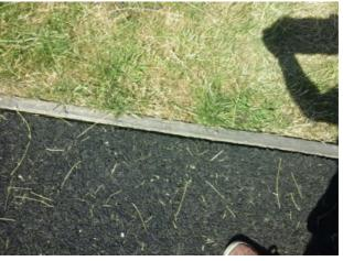
Finding: There are gaps opening between the surfacing and the edging surround or between the joints in the surfacing
