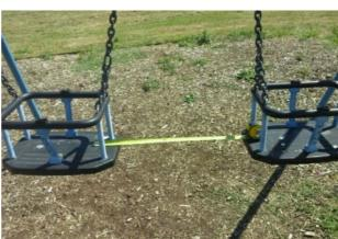
The seats are too close to each other as defined in BS EN 1176 Part 2; this is a low risk failure and no remedial action is required Finding:
