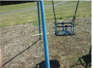
The seats are too close to the frame as defined in BS EN 1176 Part 2; this is a low Finding: risk failure and no remedial action is required
