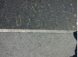
There are gaps opening between the surfacing and the edging surround or between the joints in the surfacing Finding:
