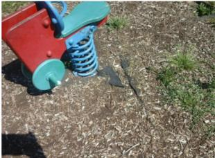
Finding: The safety surface is low and the membrane is exposed creating trip points
