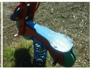
Finding: The seat is loose Action: Re secure seat
