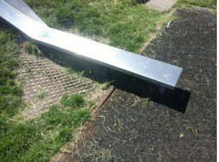
The timber edge forms a hard object within the falling space of the equipment in contravention of the requirements of BS EN Finding:
