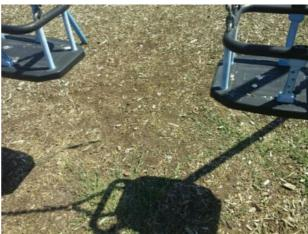
The level of loose fill surfacing has fallen significantly below the minimum 200mm recommended by BS EN 1176 Part 1 Finding:
