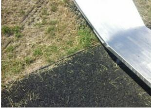
The timber edge forms a hard object within the falling space of the equipment in contravention of the requirements of BS EN Finding:
