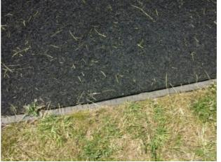
Finding: There are gaps opening between the surfacing and the edging surround or between the joints in the surfacing
