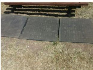
Reinstate surrounding surfaces to level to remove the trip points Finding: There are trip hazards present Action:
