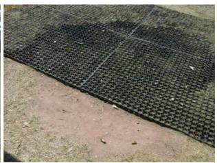
The edges of the grass mat surface have not been installed in accordance with the API Finding:
