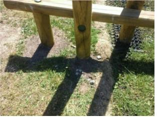
The projecting foundations forms a hard object within the falling space of the equipment in contravention of the requirements of BS EN 1176 Part 1 Finding:
