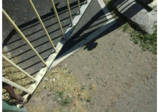
The area under the gate has eroded leaving uneven areas, or the concrete foundations Finding:
