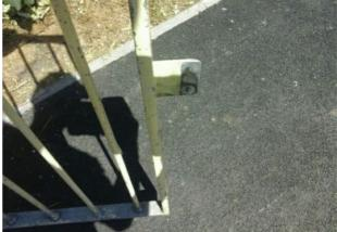
The rubber buffer is missing from the latch Finding:
