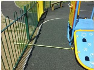
The fence forms a hard object within the falling space of the equipment in contravention of the requirements of BS EN 1176 Part 1 Finding:
