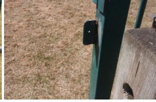
Finding: The rubber buffer is missing from the latch Action: Replace rubber buffer
