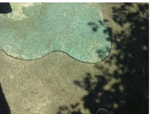
There are gaps opening between the surfacing and the edging surround or between the joints in the surfacing Finding:
