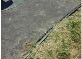
Finding: The surface is lifting at the edges and creating trip points
