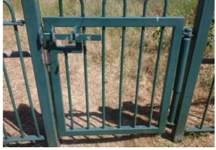
Finding: The gate is closing too quickly (less than 4 Action:
