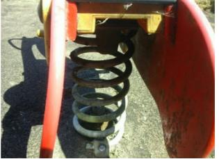
Finding: The paintwork on the spring has been damaged or worn exposing the metal underneath which is rusting
