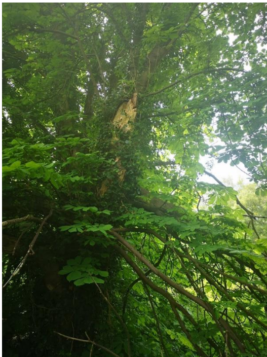
Figure 2. T33 – failed limbs
