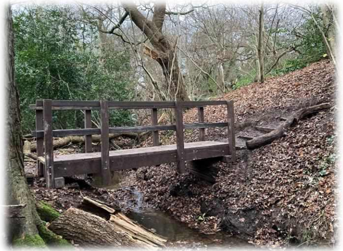
New long-lasting bridge in Hob Hey
