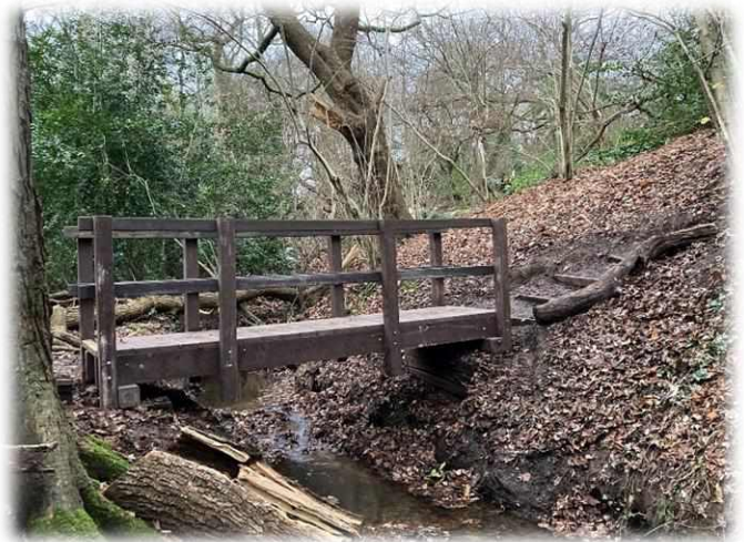
New long-lasting bridge in Hob Hey
